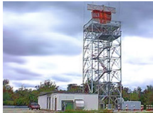
Figure 1. ASR-9 radar tower
