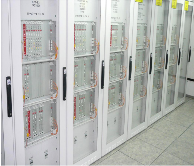
ESFAS Digital Racks (Left) and ESFAS 2 Control Systems (Right)
