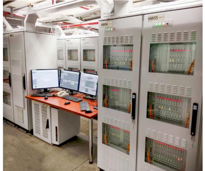
ESFAS Digital Racks (Left) and ESFAS 2 Control Systems (Right)
